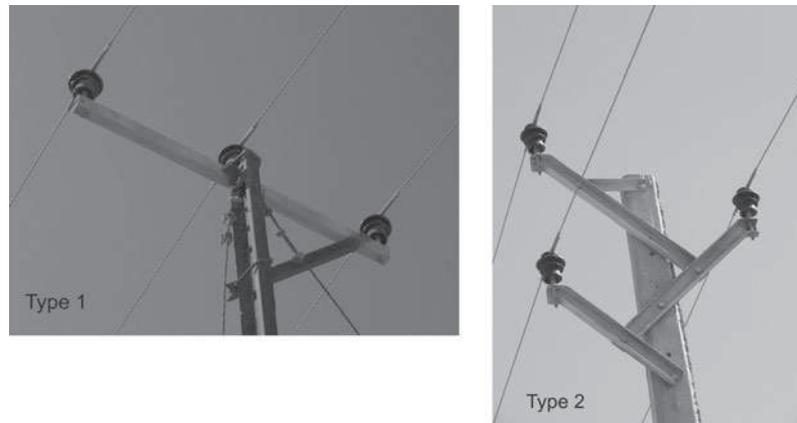
Figure 2. The two types of poles used in the powerline connecting Port Sudan and the reservoir in the area of Khor Arba'Attubular. Type 1 - rail steel poles with a T-structure supporting the conductors above the horizontal cross-arm; Type 2 - tubular concrete poles with three lateral steel cross-arms inclined at 45° and attached to the pole at different height on alternating sides.
